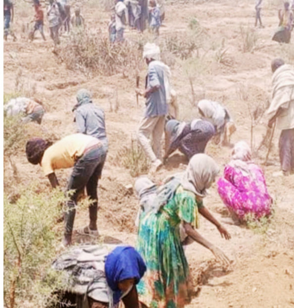
Building trenches to preserve water and prevent soil erosion.
